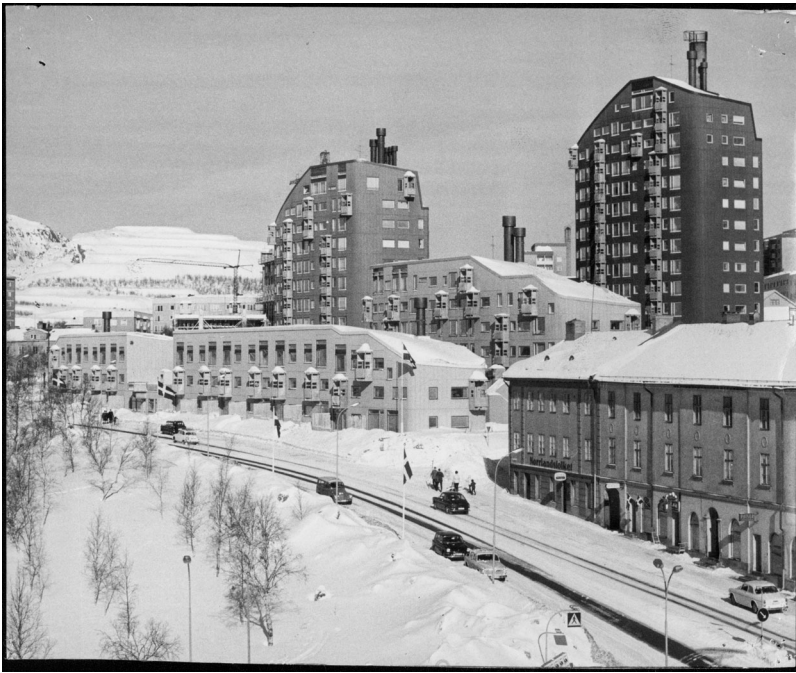
Figure 4. Ralph Erskine. Ortdrivaren quarter, Kiruna, 1959–62. View from the south-west after completion. From ArkDes Collections (ARKM.1986-122-2148). Photo: Börje Rönnberg.
