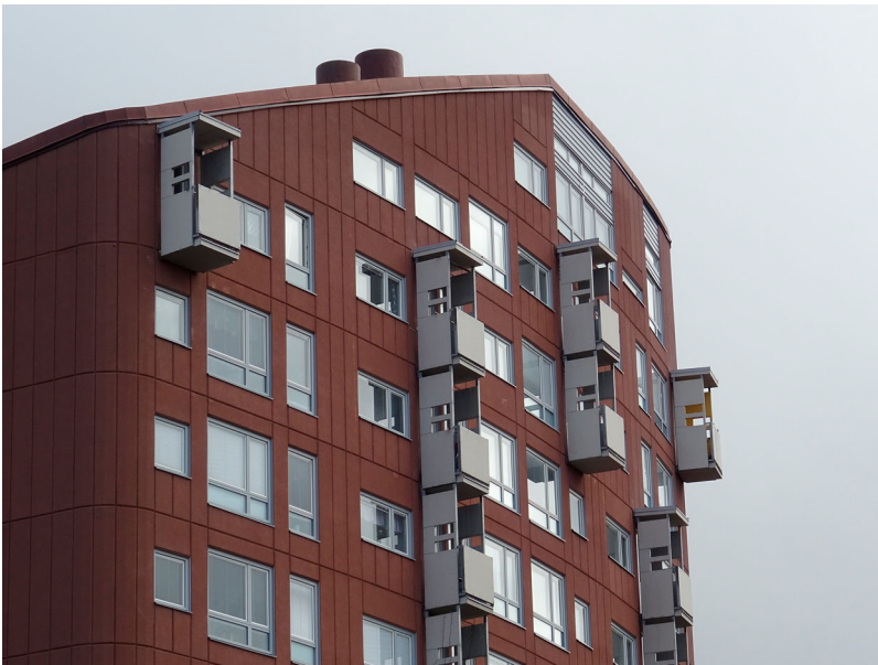
Figure 16. Ralph Erskine. Ortdrivaren quarter, Kiruna, 1959–62. Detail of the western façade of the Spottkoppfen (the original concrete balconies have been replaced), 2021. Photo: Elena Poma.
