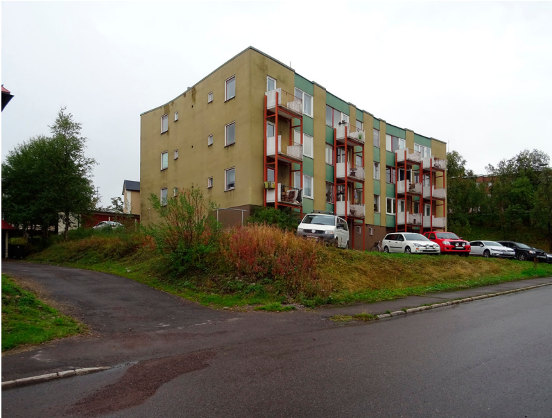
Figure 1. Ralph Erskine, apartment block in the Loket quarter, Kiruna, 1955. Exterior view from the south-west, 2021. Photo: Elena Poma.
